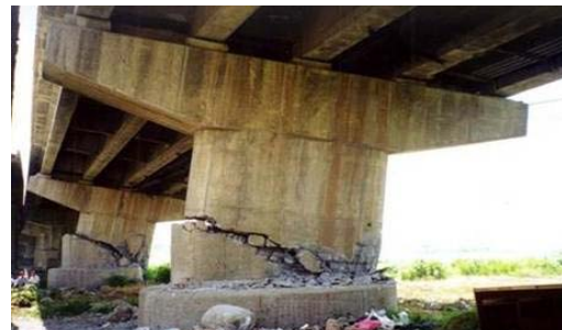
Picture 1.1 Damaged bridges in Chi-Chi earthquake
