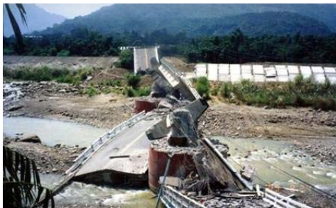
Picture 1.1 Damaged bridges in Chi-Chi earthquake
