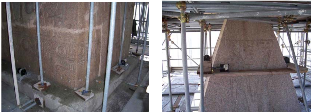
Figure 2 – Sensors on the basement and at the top of the Obelisk
