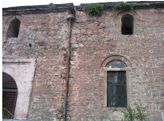
Figure 2 Cracks and damages in the walls of the mosque
