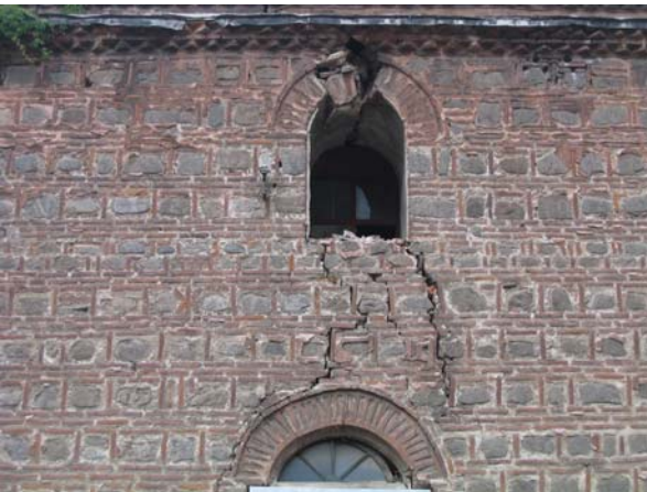
Figure 2 Cracks and damages in the walls of the mosque
