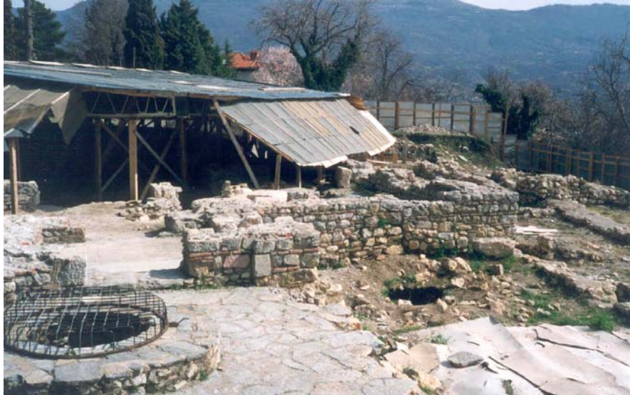
Figure 2. Existing state of the church (excavated material - 2001)
