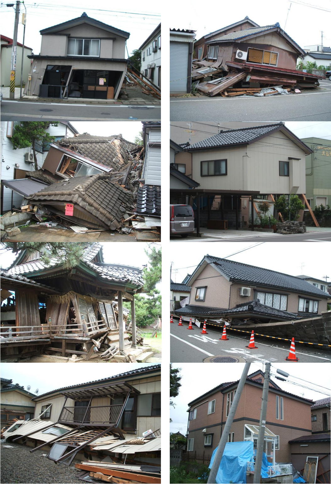
Photo 1 Damage to wooden houses due to the 2007 Niigata-ken Chuetsu-oki earthquake in Japan
