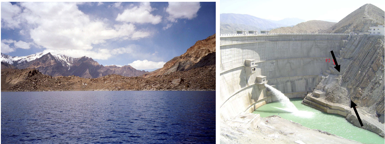
Fig. 1: Usoy dam in Tajikistan created by landslide triggered by magnitude 7.3 earthquake in 1911 (left) and arch dam in Iran with fault crossing the left abutment (right)
