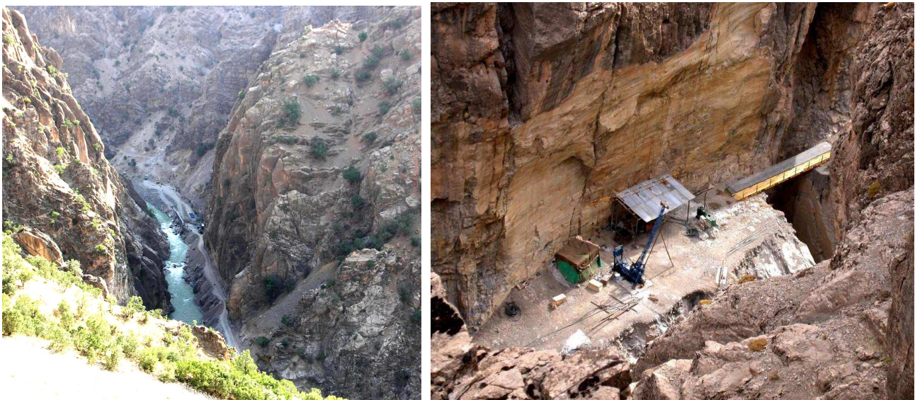
Figure 1: Rudbar Lorestan dam site in Iran: View from downstream to narrow gorge of dam site (left) and fault surface (F1) perpendicular to dam axis at left abutment during excavation of access road (right)
