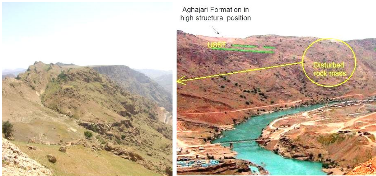
Figure 2 Right Bank, downstream view (RIGHT) and view of the upper right bank above the dam axis (LEFT).
