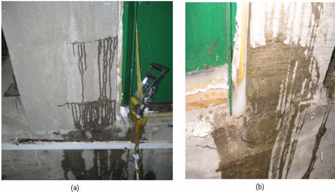
Figure 2. Experimental leakage test on wall- foundation specimens (a) wall thickness= 400mm (b) wall thickness= 300mm
