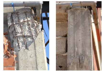
Figure 6. Column repairing
