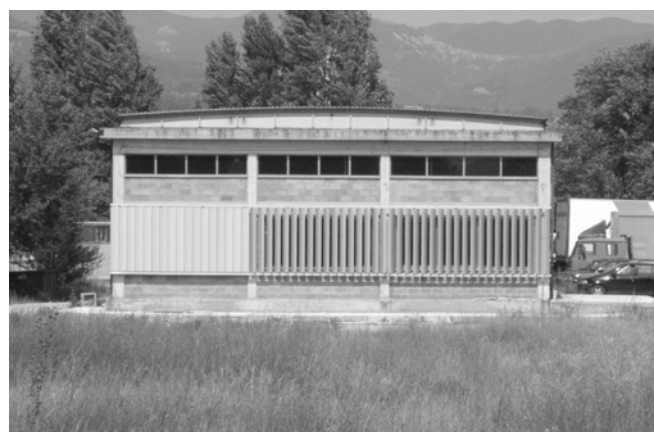
Figure 4. Typical industrial building with short elements.
