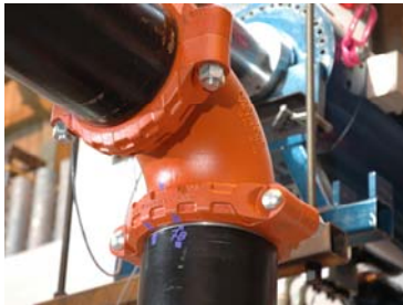
Figure 2(a) Groove coupling joint
