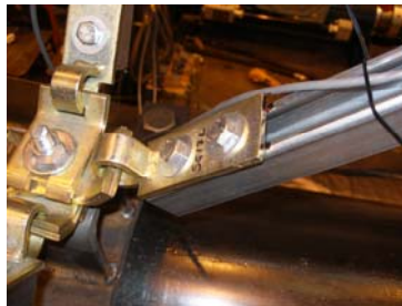
Figure 2(b) Flexible seismic bracing
