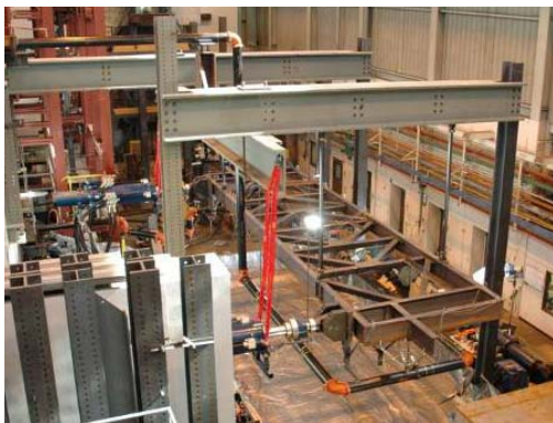
Figure 3 Photograph of loading truss
