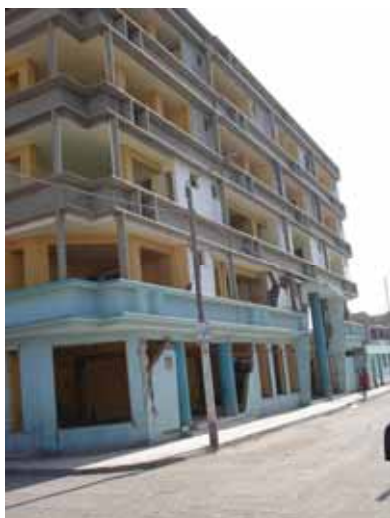
Figure 10 Reinforced concrete hotel
