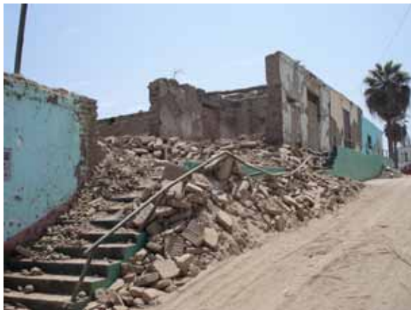
Figure 2 Collapse of adobe house
