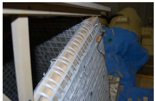
Figure 13 PP-band meshes connecting wall and roof restrain out-of-plane wall displacements
