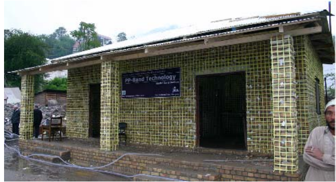
Figure 2 PP-band retrofitted house before mortar laying
