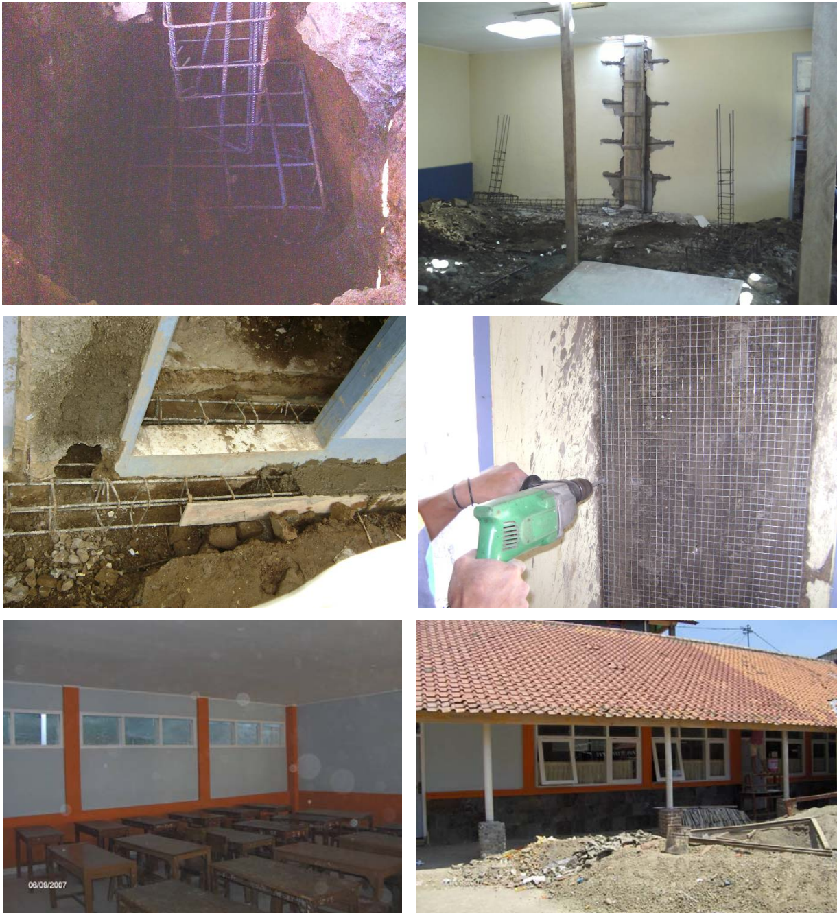
Figure 6 Various stages of the retrofitting process
