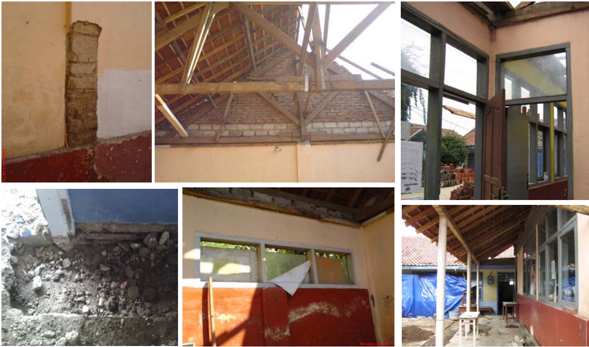
Figure 4 Existing structural condition
