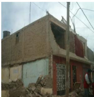
Photo 5: Overturning wall
