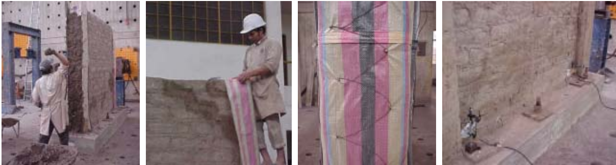
Photo 21: Four stages of reinforcement an adobe wall
