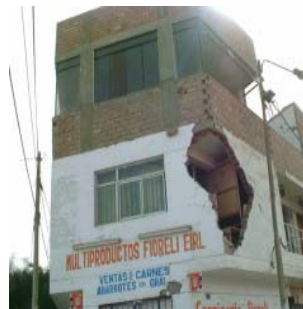
Photo 7: Facade collapse
