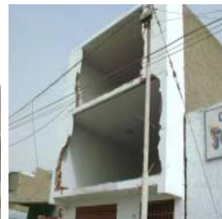
Photo 8: Collapse cantilever
