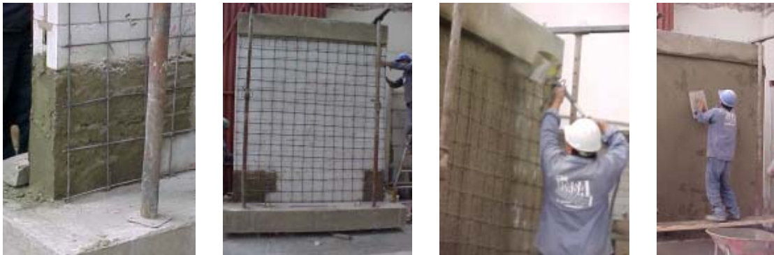
Photo 22: Four stages of reinforce a masonry wall with electro welded mesh
