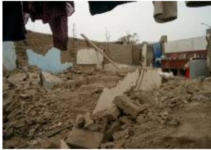
Photo 14: Total collapse on adobe house
