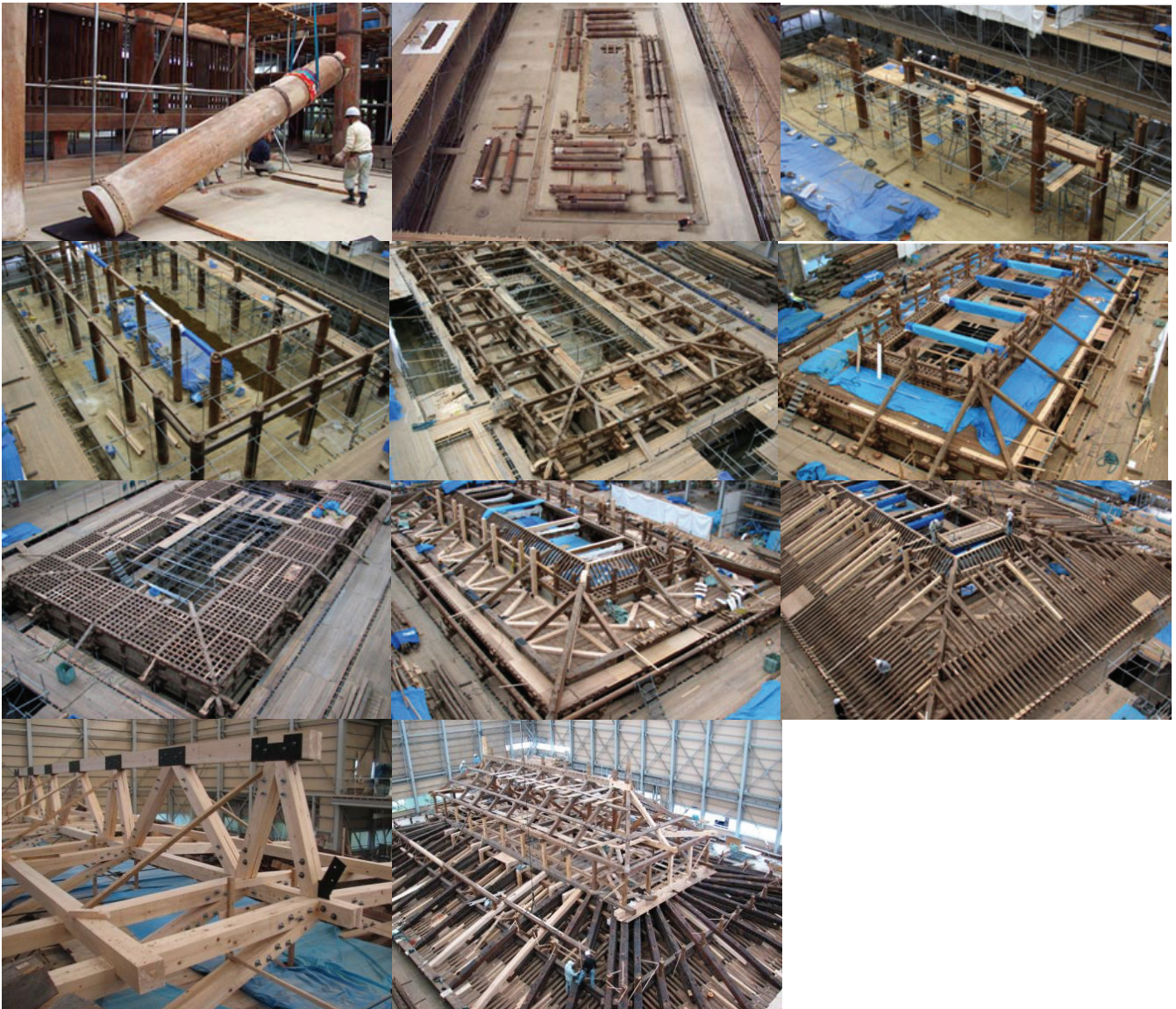
Figure 6.4 Example of repair with dismantlement(2)
