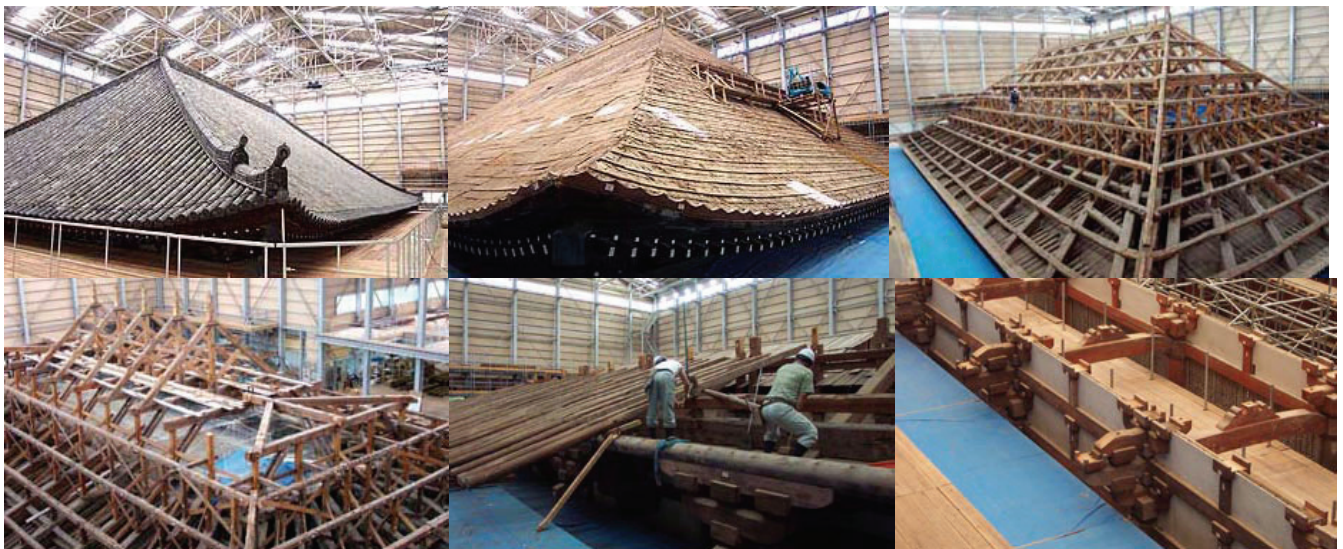
Figure 6.4 Example of repair with dismantlement(1)
