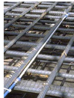
Figure 4: SOFO Sensor installed on a rebar
