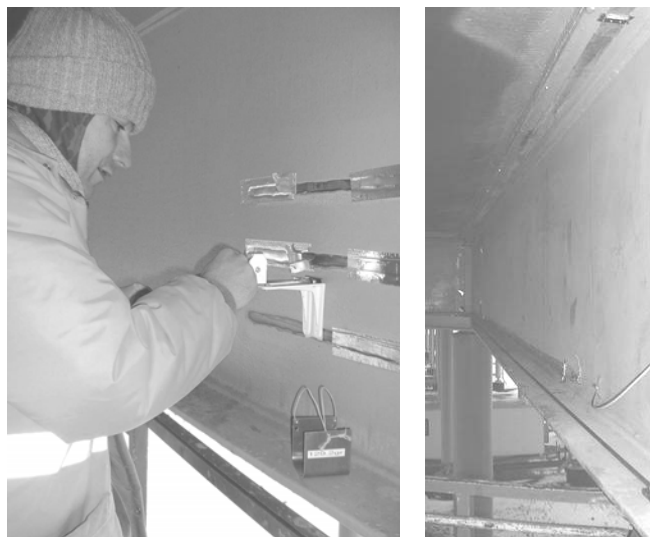
Figure 6: On-site test of SMARTape gluing procedure (left) and installed SMARTapes.
