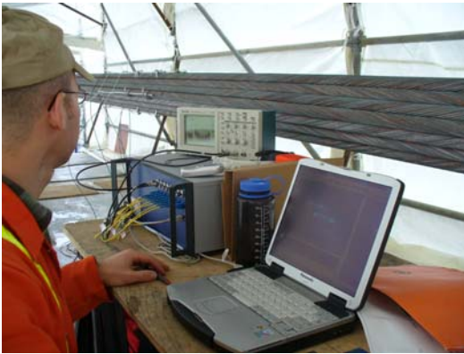
Figure 8: SOFO sensors, open cable section.
