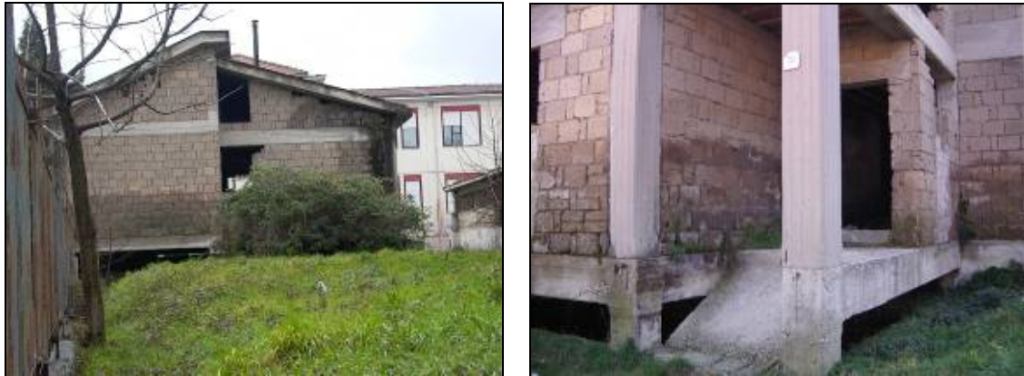
Figure 5 Existing RC framed building used a case study
