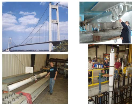
Fig 5 Jiangyin Yangtze River Bridge and dampers
