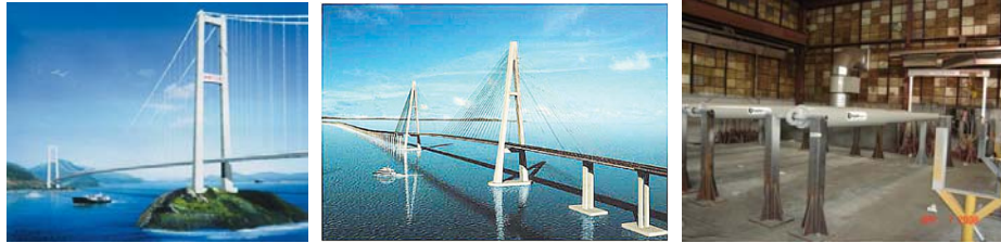
Fig 6 Xihoumen and Jingtang Bridge and dampers
