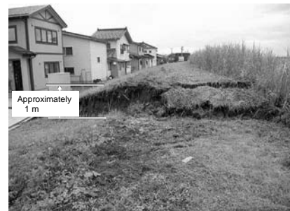
Photo 6 Subsided bank of Sabaishi River
