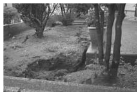
(a) Asahigaoka: Crack in the garden of a house
