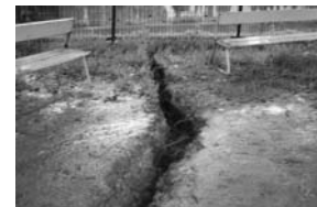
(b) Minamihanda : Crack in the ground of a park
