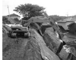
(a) Banjin 2-chome: Retaining wall bumped against front houses (Photo: By Niigata Local Government)
