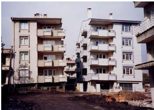
Photo 3 Two apartments tilted outside in Adapazari during 1999 Kocaeli earthquake
