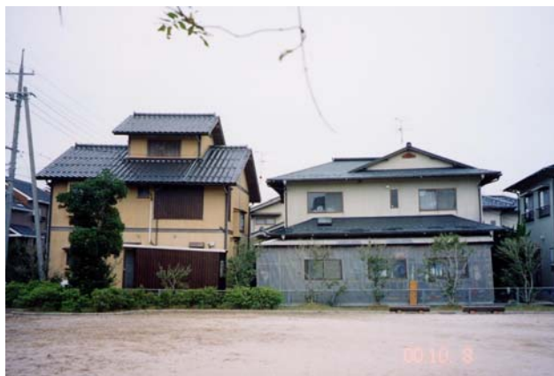
Photo 1. Settled and tilted houses due to liquefaction in Abehikona development
