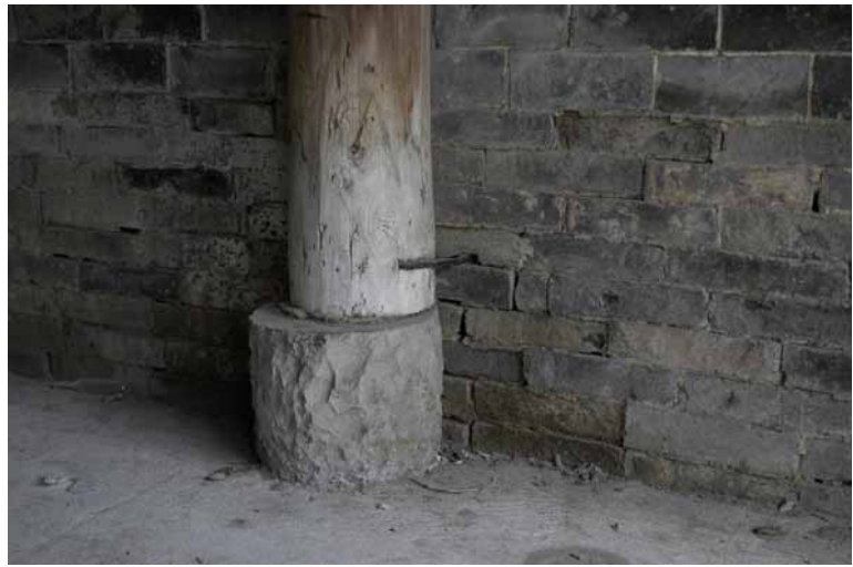
Figure 12 Brick-wood structure, Ningbo, China
