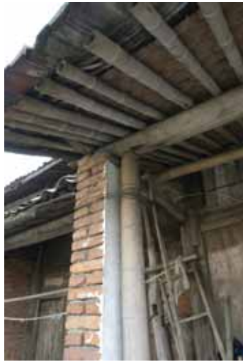
Figure 11 Brick-wood structure, Ningbo, China
