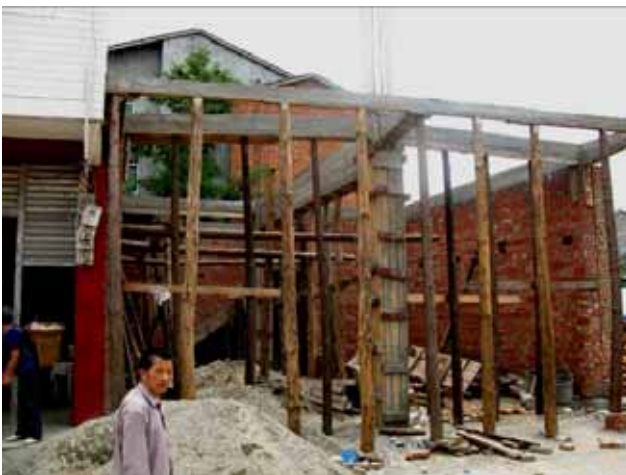
Figure 1 Brick structure, Ms 8.0 Wenchuan Earthquake
