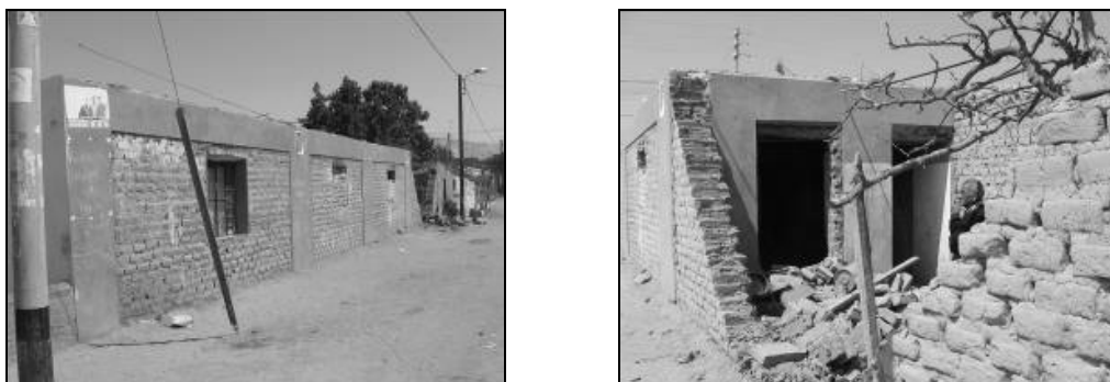
a) Reinforced building
