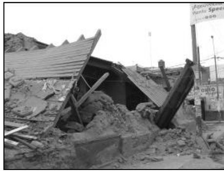
a) Plinth wall made using clay bricks
