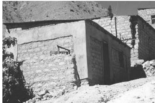
Reinforced house (Arequipa earthquake 2001)
