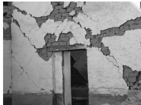
Diagonal cracks
