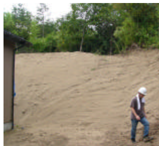
Figure 10. Liquefaction in slopes
