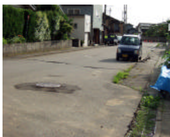
Figure 15. Differential settlement
