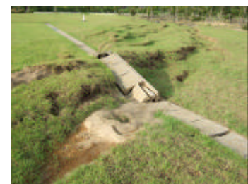
Figure 18. Uplifting due to lateral flow
