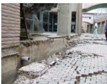
Figure 19. Entrance of the building
