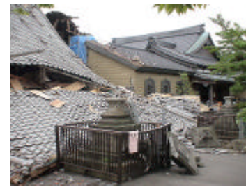
Figure 6. Damages to wooden traditional structure (Monkoji temple)
