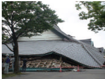
Figure 6. Damages to wooden traditional structure (Monkoji temple)
