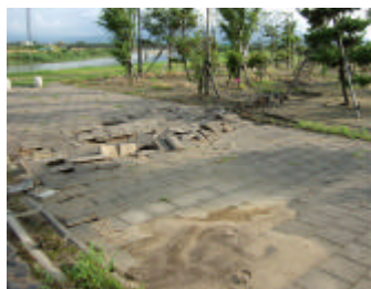
Figure 18. Uplifting due to lateral flow
