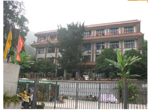
(Grade 1) Slight damage
