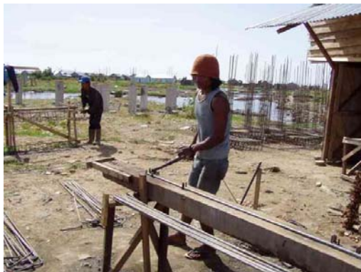
Figure12 Bending works with simple tool
