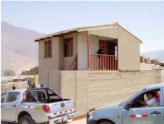
Figure3 Model House in Zuniga in Peru No structural damage by Pisco Earthquake
