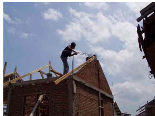
Figure13 Placing of fabricate rebar
