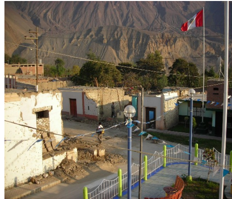
Figure4 Central part of Zuniga in Peru Many adobe houses collapsed
