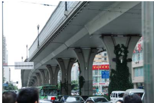
Fig.29 Viaduct at Chengdu
