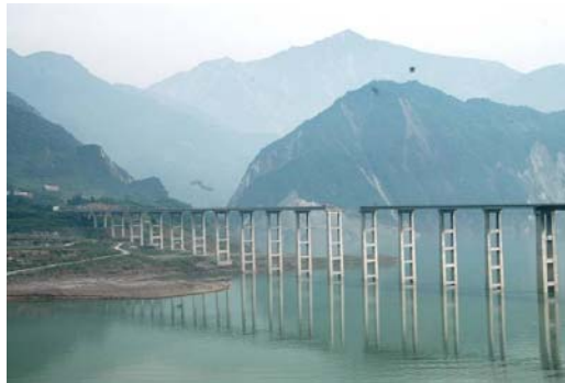
Fig.15 The approached of Miaotzuping Bridge
