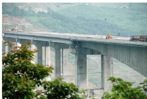
Fig.17 Horizontal shift of spans
