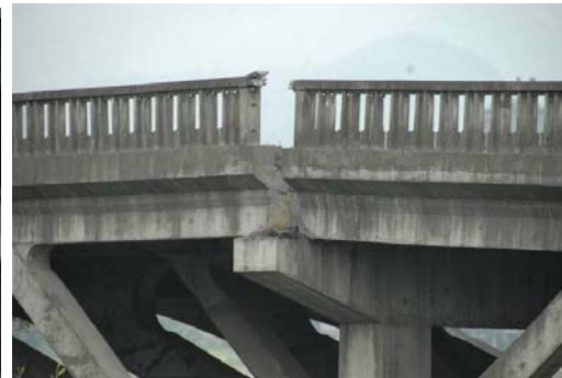
Fig. 14 Horizontal displacement of the spans
