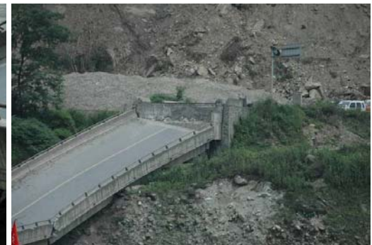
Fig.6 The abutment of Baihwa Bridge
