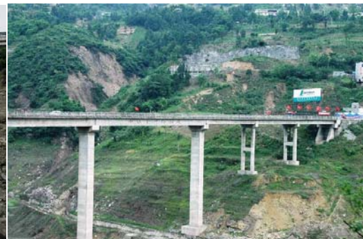
Fig.20 No damages observed on piers
