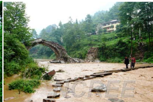
Fig.28 Damaged Bailu bridge and the emergency detour
