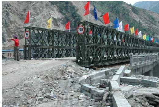
Fig.25 Bailey bridge with speed and weight limits
