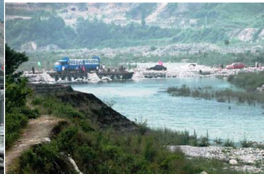
Fig.26 Emergency detour of Xiaoyudong bridge
