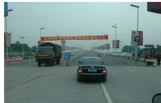
Fig.32 Warning Sign for bridge at Mianzhu
