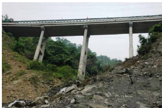
Fig.19 Horizontal shifts of the decks
