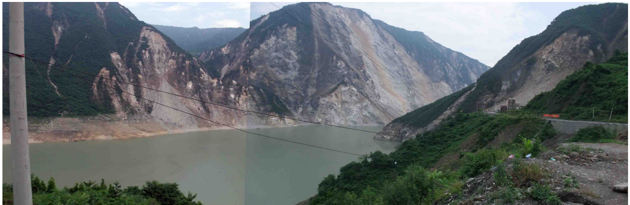
Figure 6 Coseismic fault with vertical displacement 0.5m inside tunnel BYD (middle), where located at intersection of the road in right front (bottom). The river and valley are along the NE fault near BYD as the map shown. Many land sliding occurred along steep mountains.
