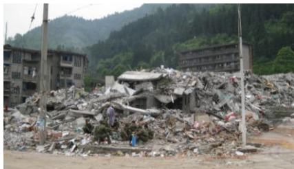
Fig. 19 Many old brick buildings collapsed
