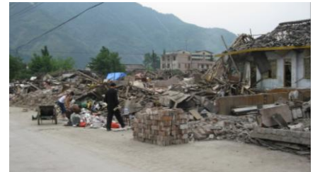
Fig. 18 Lots of old brick-wooden houses collapsed
