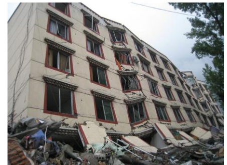
Fig. 15 A five story brick building collapsed
