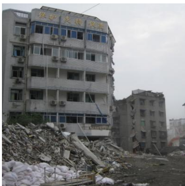
Fig.28 One side of a L-type building collapsed, now another behind damaged building can be seen
