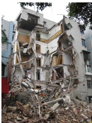
Fig. 36 Partly collapsed brick building
