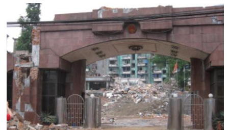
Fig. 24 All the town government buildings collapsed, only the gate left
