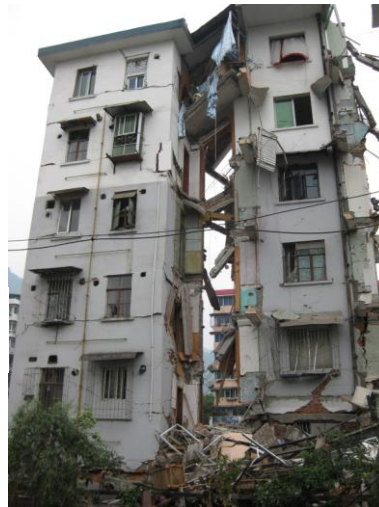
Fig. 25 Front brick-wooden houses collapsed, behind brick buildings heavy damaged
