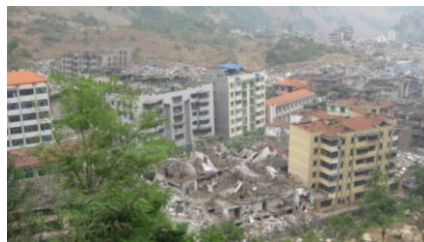
Fig. 2 Another scene of heavy damaged and collapsed buildings
