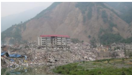
Fig. 1 Heavy damaged and collapsed buildings
