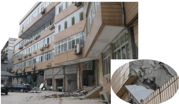
Fig.34 First story damage of a five story frame building with local enlargement of one node of column and beam
