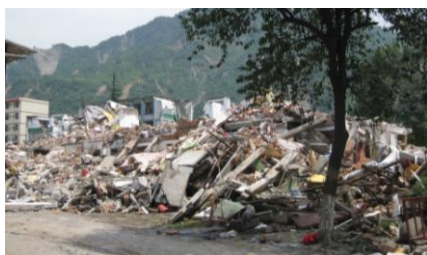
Fig. 22 Many brick buildings collapsed
