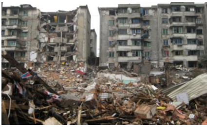
Fig. 25 Front brick-wooden houses collapsed, behind brick buildings heavy damaged
