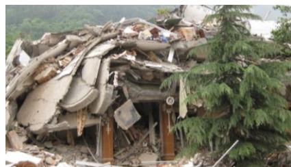
Fig. 8 Upper stories of BBF building collapsed
