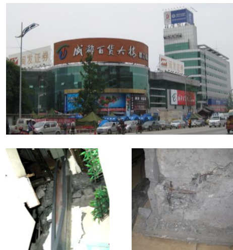
Fig. 35 Damage of a frame and frame-shear wall united building
