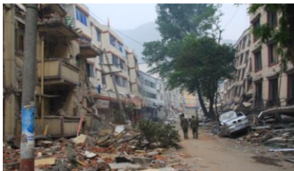
Fig. 13 All the buildings collapsed or heavy damaged along the street
