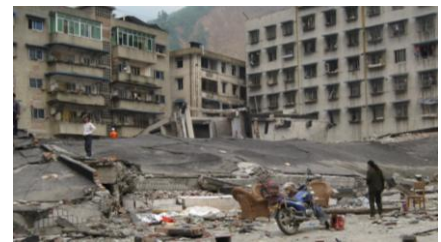
Fig. 3 Front building collapsed; behind-left building heavy damaged, behind-right building slight damaged
