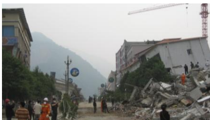
Fig. 7 All the buildings collapsed or heavy damaged along the street
