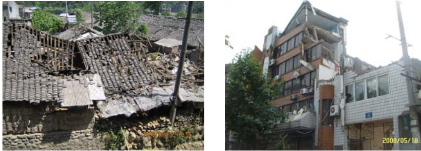
Figure 9 Severe damages of countryside house and buildings without seismic protection
