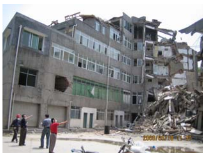
Figure 14 Severe damage of buildings with elevation irregularity
