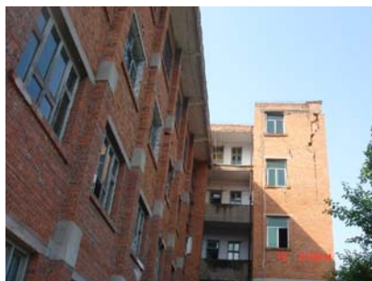
Figure 13 Severe damage of buildings with plane irregularity
