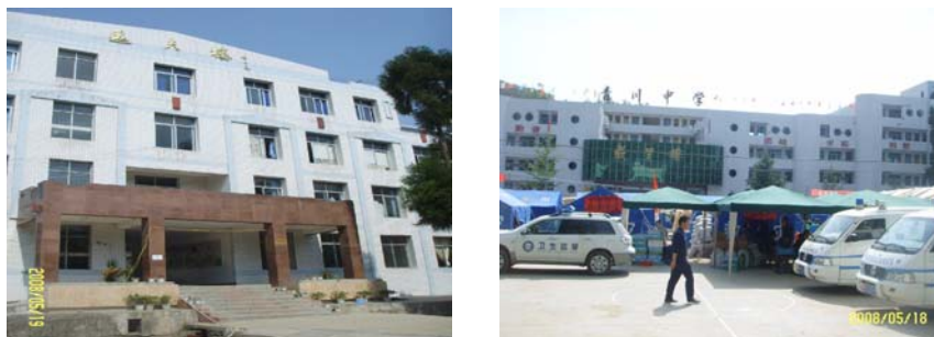
Figure 10 Slight damages of teaching building of two schools
