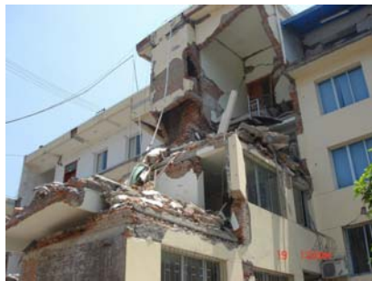
Figure 6 Severe damage of stair part due to irregular plane (T-shaped)
