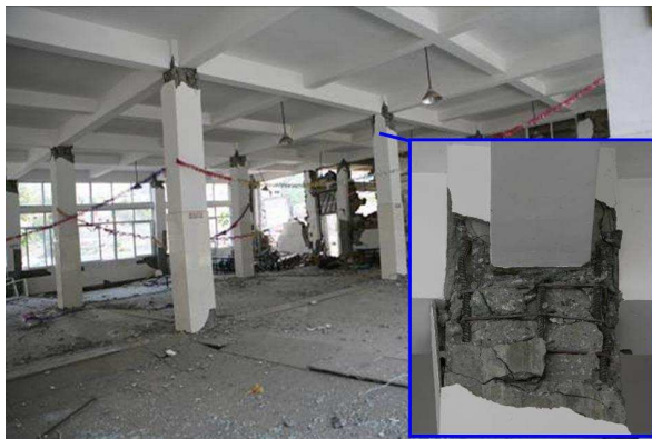
Figure 2 Plastic hinging in columns
