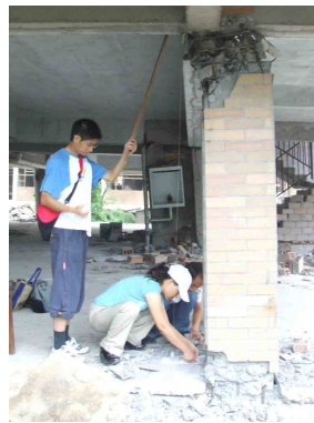
(b) Measuring column drift
