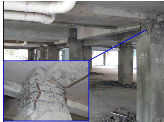
Figure 3 Weak-column and strong-beam
