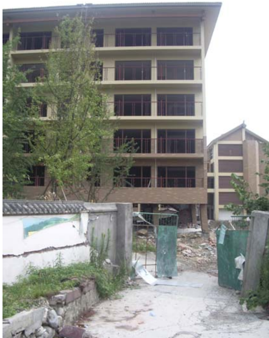
Figure 4: Six-storey RC MRF in Yazhouyan housing development, Dujiangyan that is exhibiting a soft-storey failure mechanism at ground storey (detail of ground floor columns, right)
