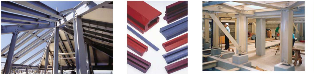
Figures 6, 7 & 8 – Examples of high strength FRP applications in building construction (Courtesy photos from Strogwell Corp., Bristo, VA)
