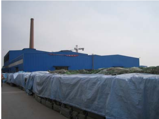
Figure 10 the whole building of Hung-sen Glass Co.
