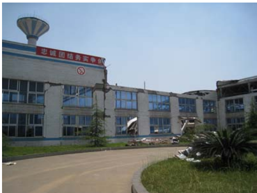
Figure 8 the whole building of Xiting Packing Co.
