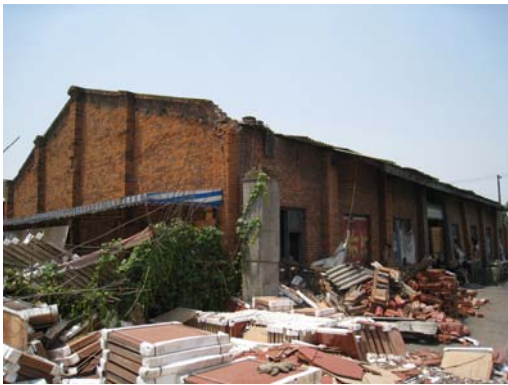
Figure 6 the whole building of Mianzhu marble factory
