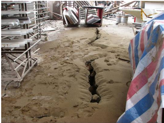
Figure 4 Liquefaction-induced destruction to factories (Photo by N. Gao)
