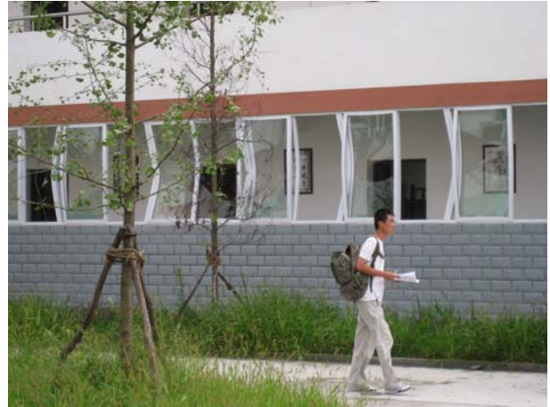
Figure 2 Liquefaction-induced settlement/differential settlement in Wenchuan Earthquake (Photo by L. Chen)
