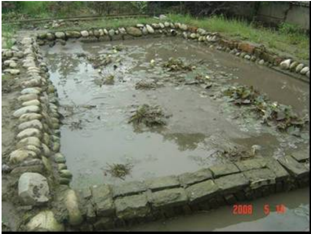
Figure 7 Liquefaction-induced destruction to fishpond and swimming pool (Photo by E. Guo and Z. Cao)
