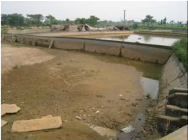
Figure 6 Liquefaction-induced destruction to aqueduct and reservoir (Photo by Z. Cao)
