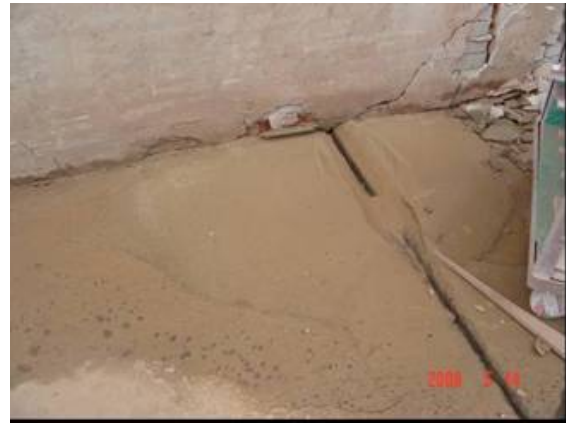
Figure 4 Liquefaction-induced destruction to factories (Photo by N. Gao)
