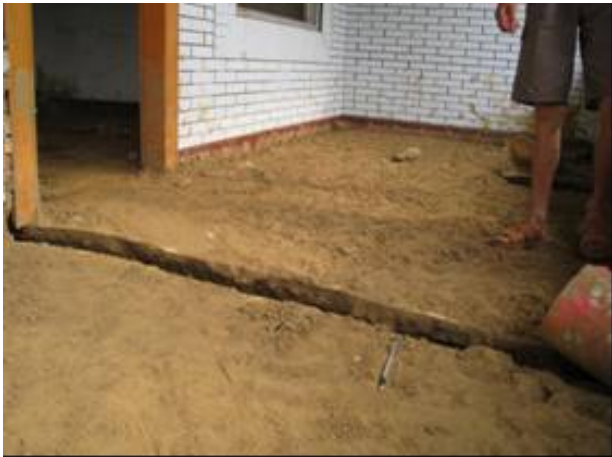
Figure 5 Liquefaction-induced destruction to residences (Photo by Z. Cao)
