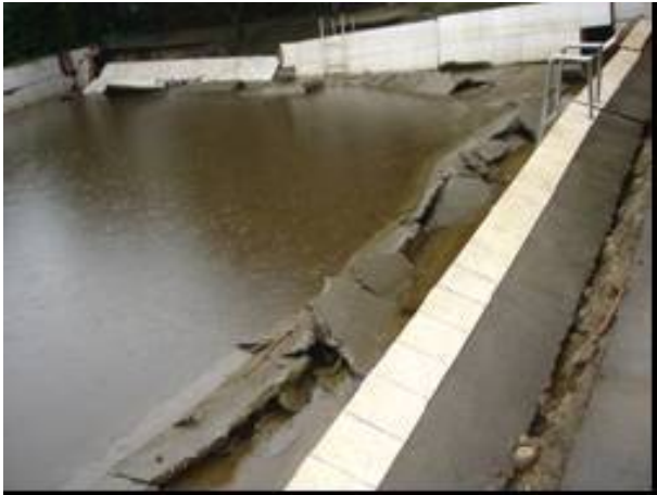
Figure 7 Liquefaction-induced destruction to fishpond and swimming pool (Photo by E. Guo and Z. Cao)
