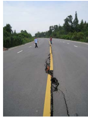
Figure 3 Liquefaction-induced destruction to bridge and road (Photo by Z. Cao and F. Meng)
