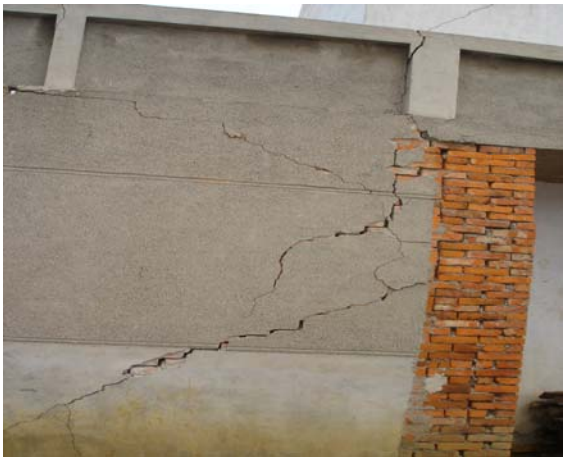
Figure 5 Liquefaction-induced destruction to residences (Photo by Z. Cao)
