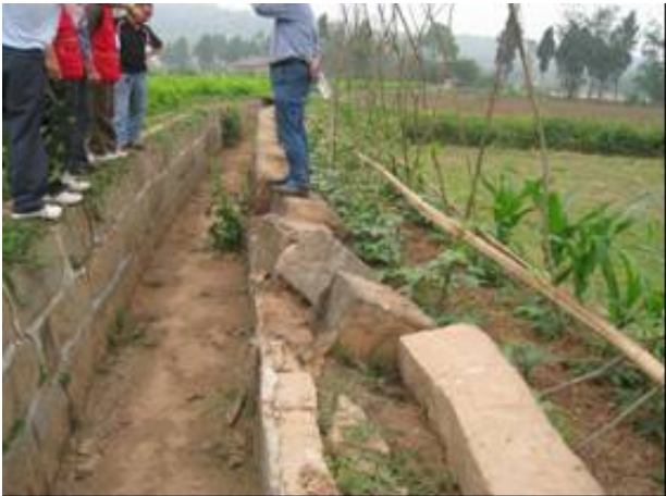
Figure 6 Liquefaction-induced destruction to aqueduct and reservoir (Photo by Z. Cao)
