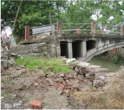
Figure 3 Liquefaction-induced destruction to bridge and road (Photo by Z. Cao and F. Meng)
