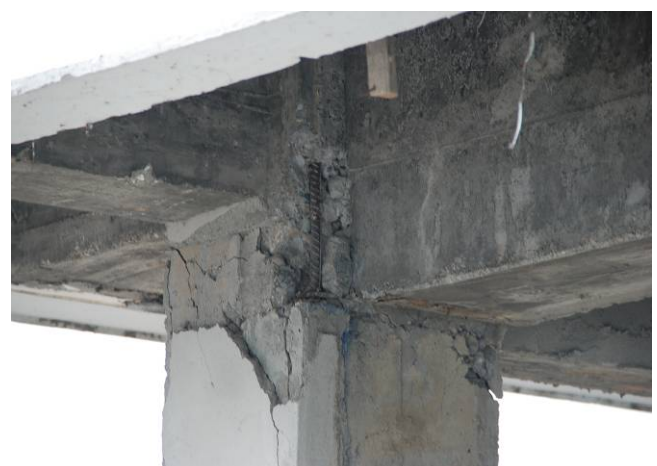
Fig.8 Top story damage
