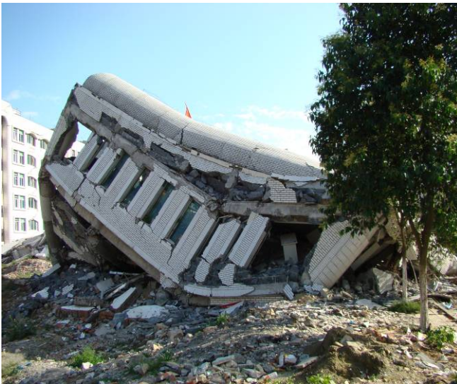
Fig.12 collapse of a 9-story frame building
