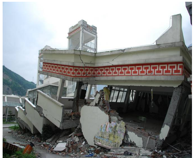
Fig.13 collapse of a 4-story frame building
