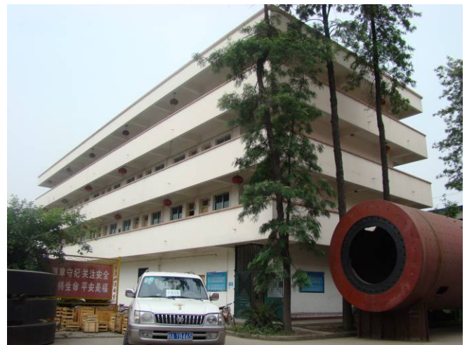
Fig.2 4-story office building of Chuankuang Group
