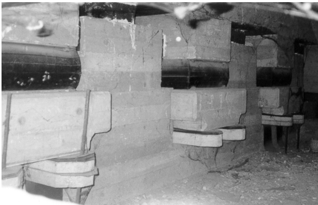
Figure 1. Rubber bearings placed between the strip foundation and the building
