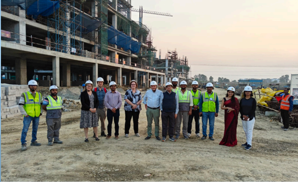
A group of faculty from The University of Melbourne visited the GSMST construction site.
