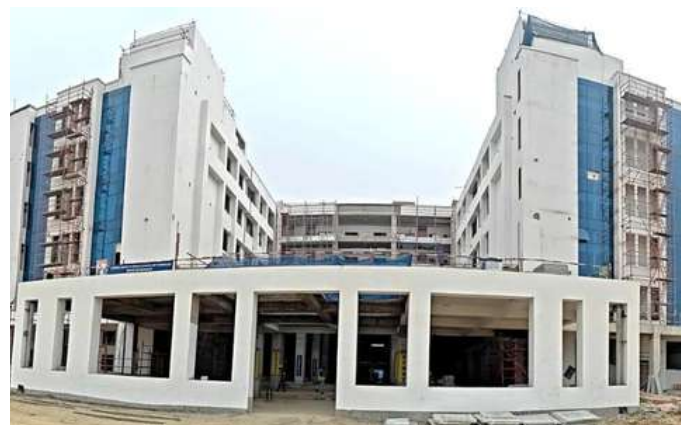
Current view of the GSMST construction site
